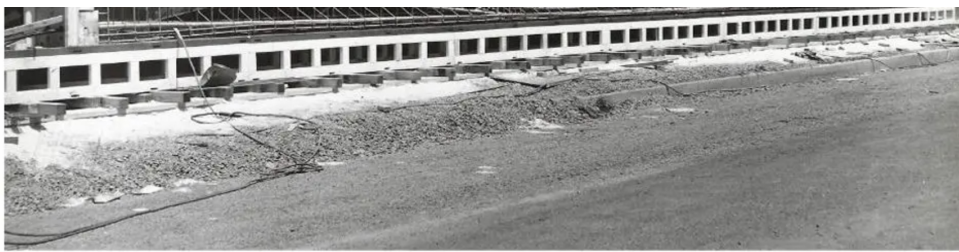
Post-Tensioned, Prestressed, Precast Beam for the Gettysburg College Dining Hall circa 1958
